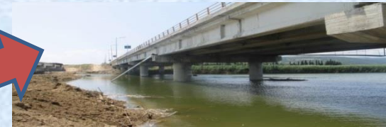
V3: Strymonas river bridge, Egnatia Odos, September 2018
